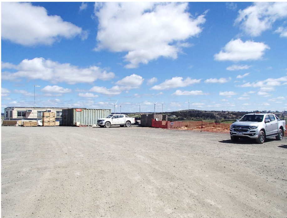
Plate 4 Typical contractors site office and amenities compound
