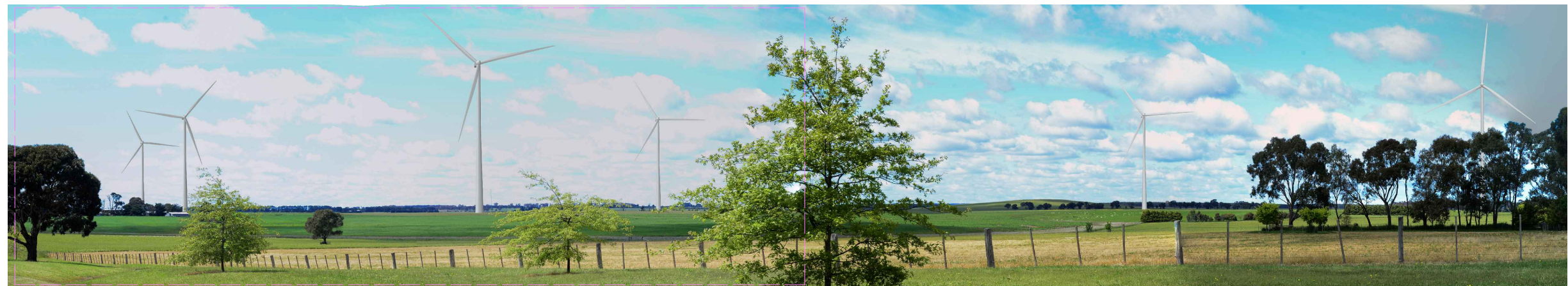
Photomontage P10 - Proposed view north east to south east from Pin Oak Court. Approximate distance to closest visible wind turbine (T5) 1.13km
