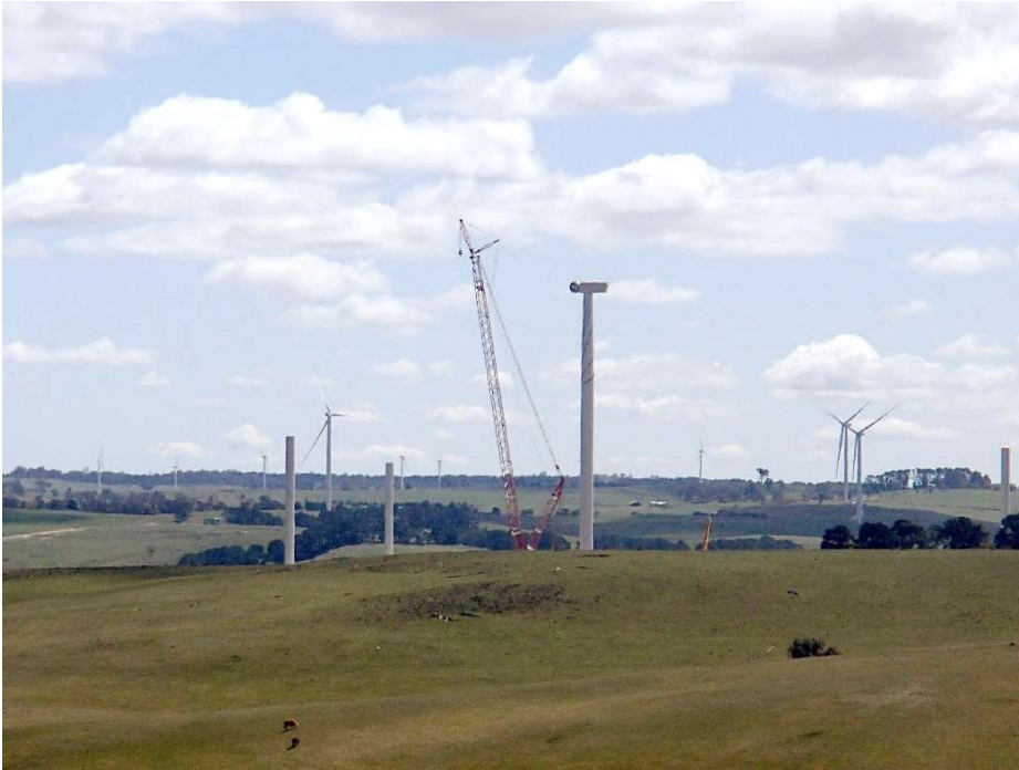
Plate 5 Typical view toward wind turbines under construction
